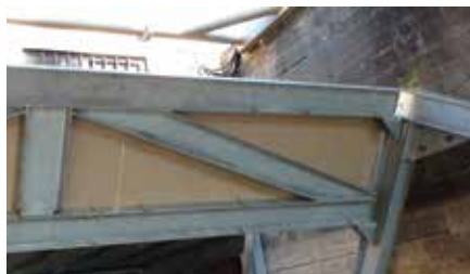
Welded Steel supporting structure
