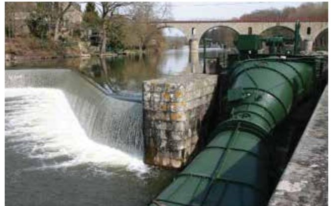
Typical layout of an existing Mayenne HPP with a Siphon Kaplan installed in parallel with a navigation lock
